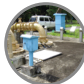
Drilling and Well
